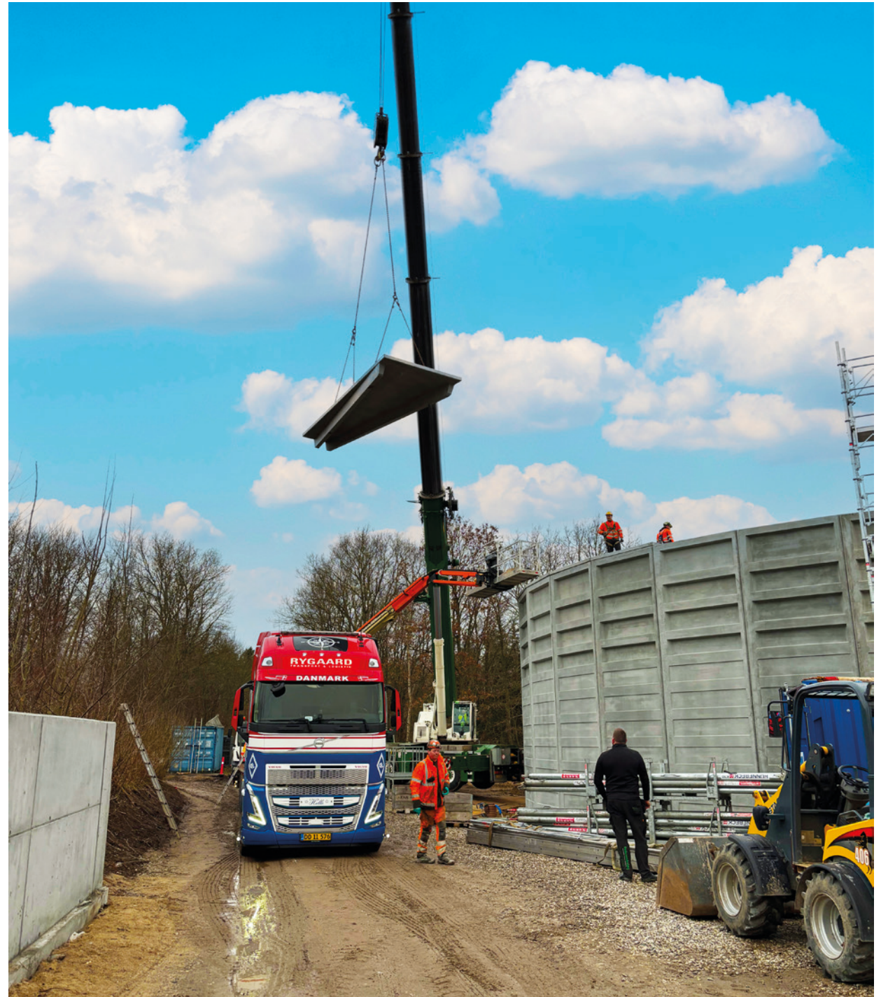
Construction of a new wastewater tank at the SecAnim plant, increasing the wastewater treatment capacity.
